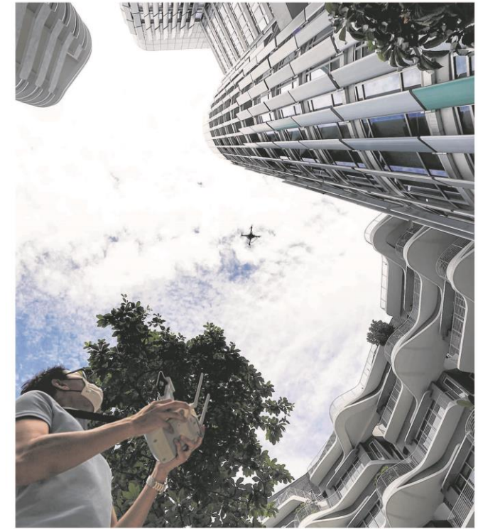
Equipped with high-resolution cameras, drones are used to scan the hospital buildings' exterior and can capture live footage of hard-to-reach areas such as roof gutters, and detect water ponding on rooftops. ST PHOTO: KELVIN CHNG
